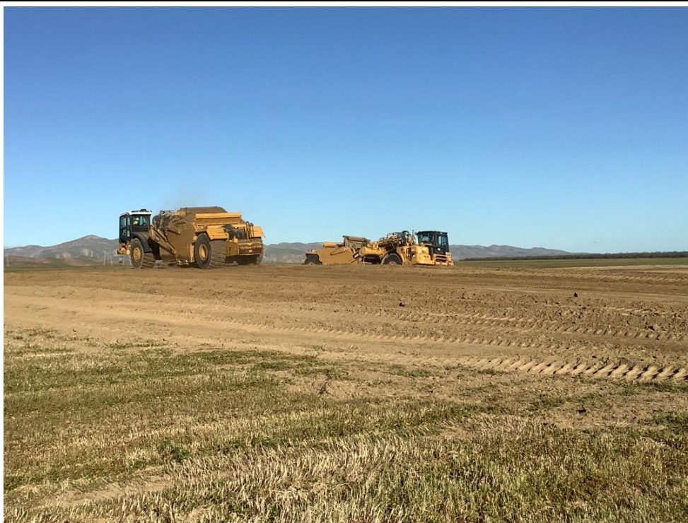
Photograph 4: CBI crew using scrapers to stockpile topsoil on 3/2/2026.
