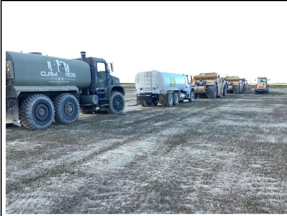
Photograph 5: Vehicles in place with secondary containment at end of day on 3/4/2026.
