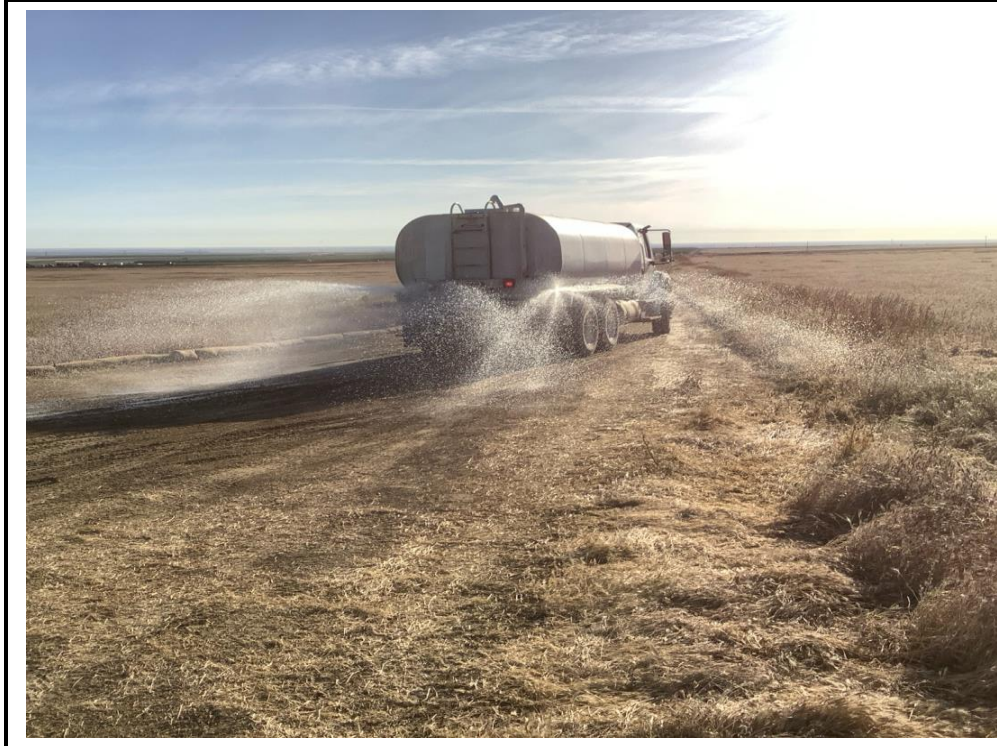
Photograph 7: Water truck spraying water on access roads to mitigate fugitive dust on 3/16/2026.
