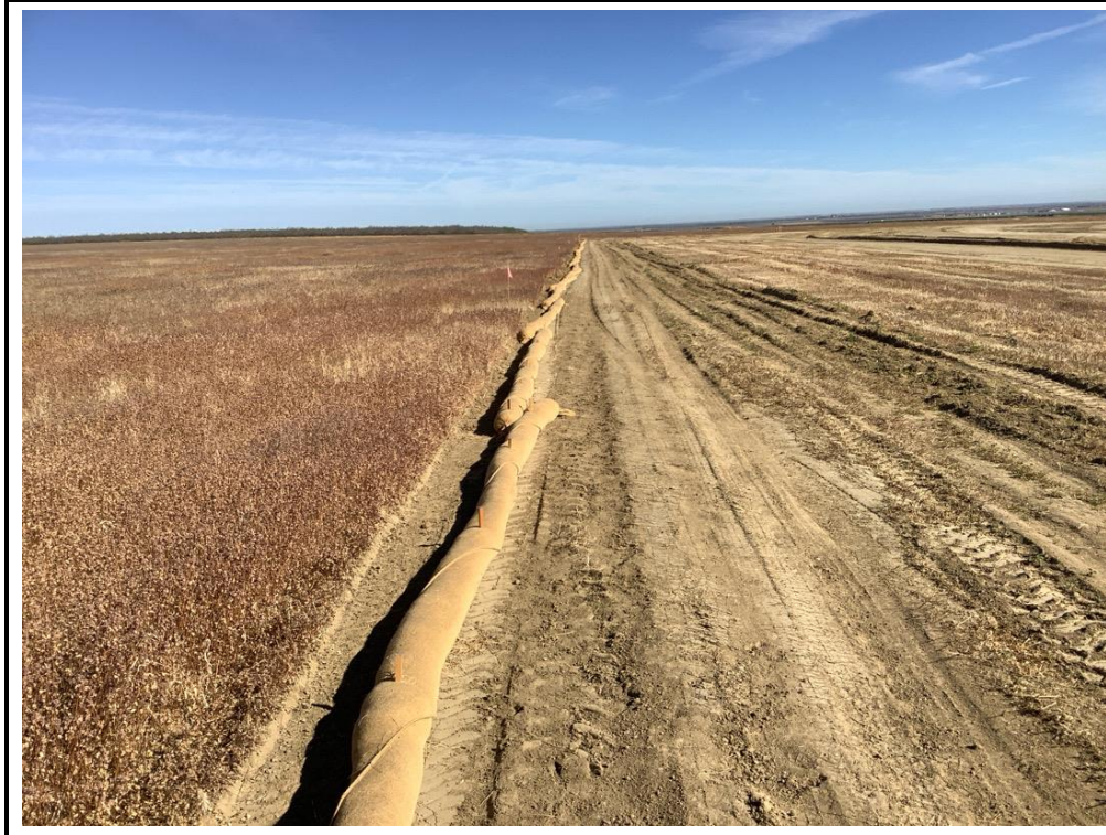
Photograph 9: Straw wattle BMP in place along access road on 3/25/2026.
