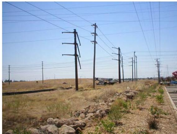
Figure 2-6. Pole installations north of the Atlantic Substation; the side arms were later erected just prior to stringing operations
