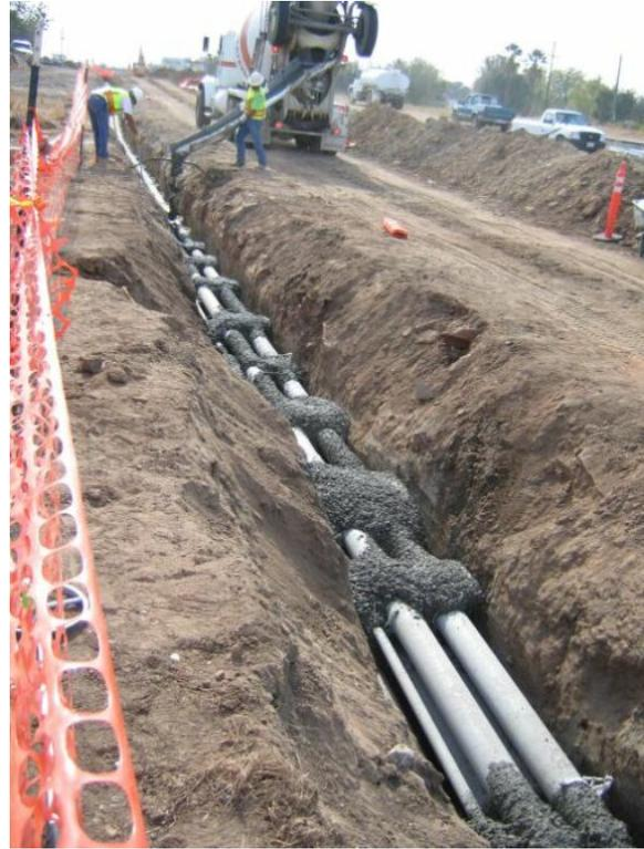
Figure 2-12. Thermal concrete pour over conduit installation north of Farron Road
