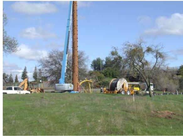
Figure 2-26. Transition Pole #10 and conduit stringing operations at Vault #1
