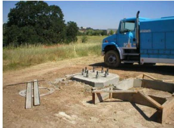
Figure 2-2. Completed foundation base at Pole #17
