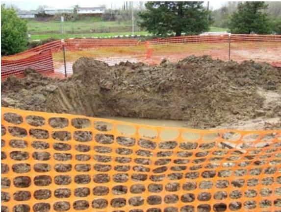
Figure 2-25. Detention pit used for dewatering
