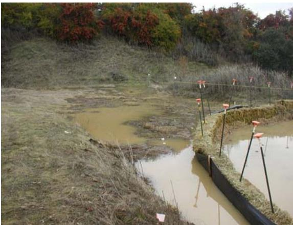
Figure 2-27. Sediment-laden runoff into Wetland #2
