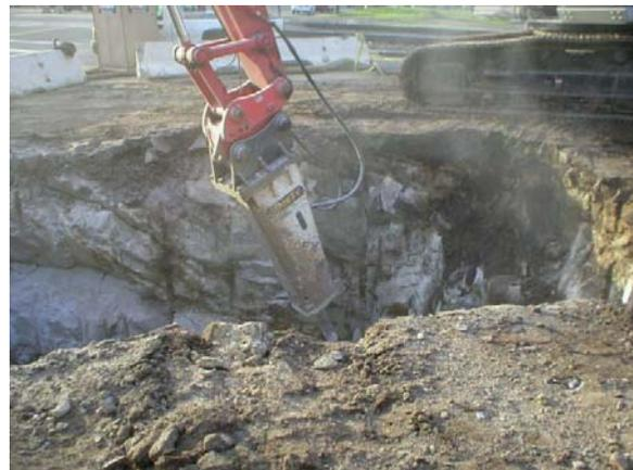
Figure 2-14. Rock hammering at Vault #3
