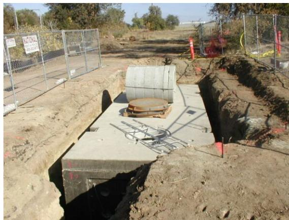
Figure 2-18. Vault #4 installation
