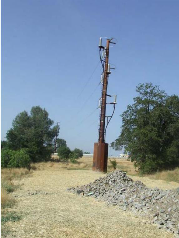
Figure 2-9. Completed Transition Pole #9
