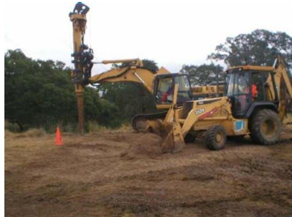
Figure 2-4. Auger of the foundation hole for Pole #20
