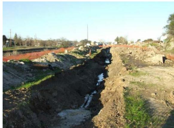
Figure 2-17. Excavation and conduit installation north of Rocklin Road
