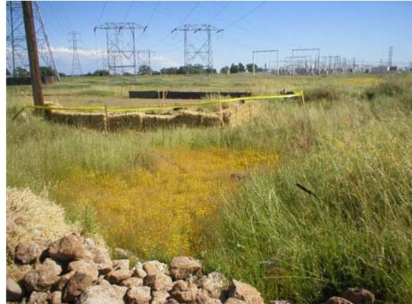
Figure 2-3. Vernal pool area (foreground) protected by installed erosion controls surrounding Pole #4
