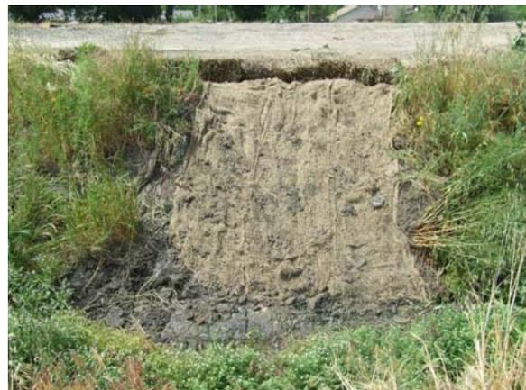
Figure 2-24. Final repair of Drainage #30
