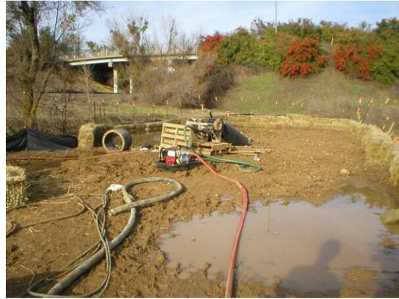
Figure 2-33. Dewatering the bore pipe into Wetland #2
