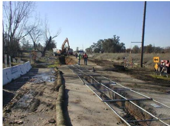
Figure 2-13. Trenchline excavation and conduit installation
