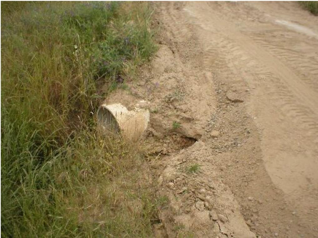
**Figure 2** – Fine dirt created after grading over the access road drainage near Pole 2/16, May 17, 2005.
