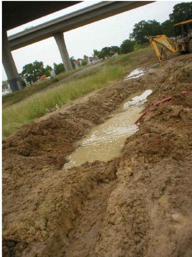
**Figure 6** – Dewatering ditch created to contain groundwater from the Pole 2/15 foundation hole, May 17, 2005.
