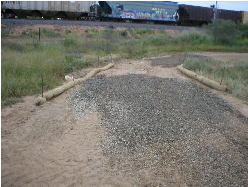
**Figure 3** – Photo after the fine dirt had been removed and replaced with clean gravel over the access road drainage near Pole 2/16, May 17, 2005.
