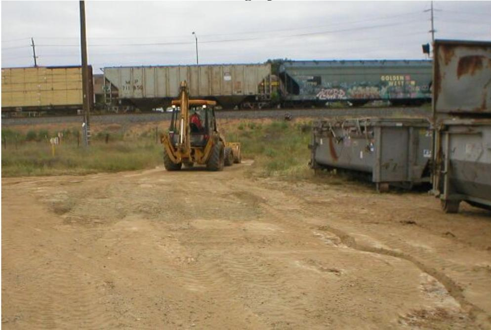
**Figure 1** – Grading over the access road drainage near Pole 2/16, May 17, 2005.
