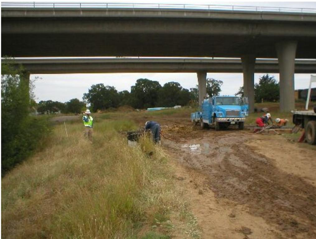
**Figure 4** – Dewatering groundwater from the Pole 2/15 foundation hole, May 17, 2005.
