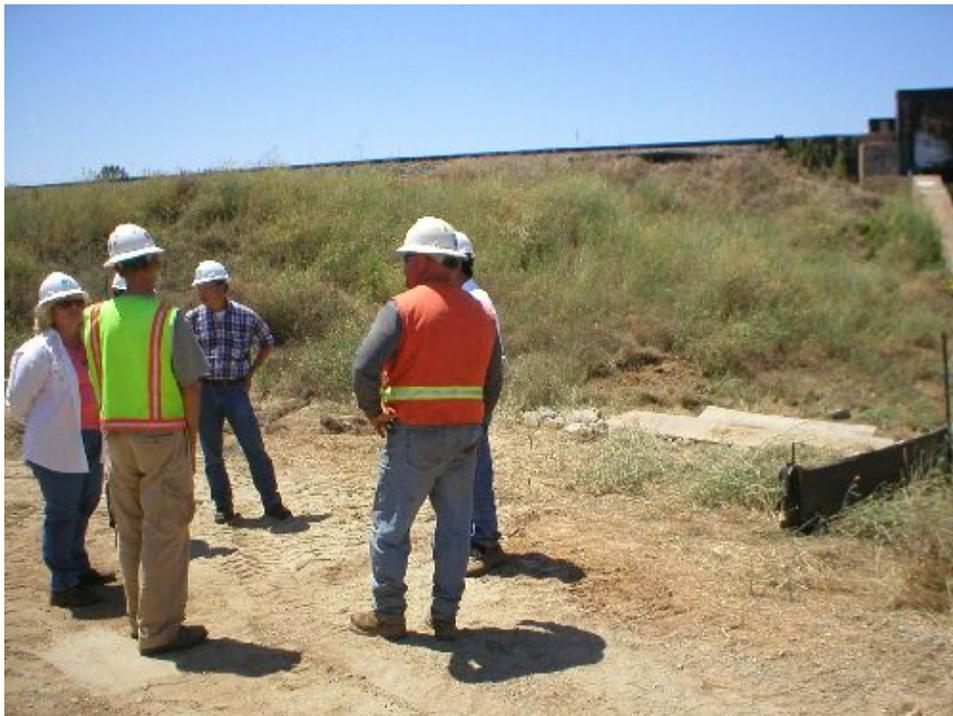
**Figure 2** – Crew Forman, PG&E engineers, and PG&E EI on-site at Pole 7 (the foundation hole is covered by wood to the right of the meeting area) to discuss feasible options to complete the foundation work due to the encountered rock, June 30, 2005.
