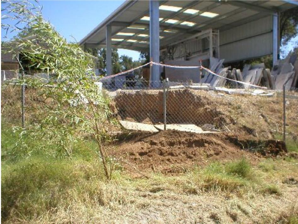
**Figure 1** – Crews covered the 10-foot deep augured foundation hole at Pole 6 adjacent to the railroad, August 6, 2005.
