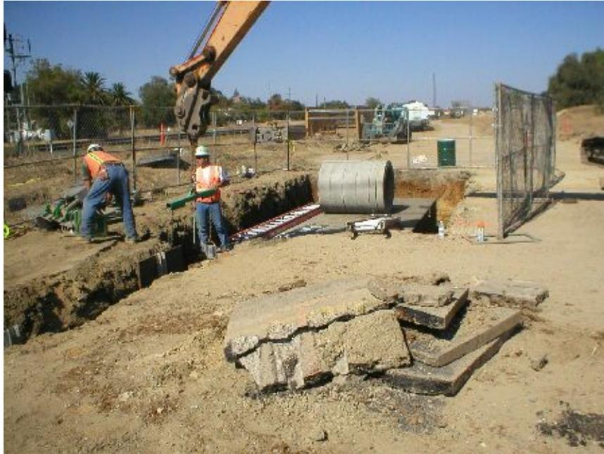
**Figure 1** – Vault installation with extending trench line north of Farron Street, September 15, 2005.
