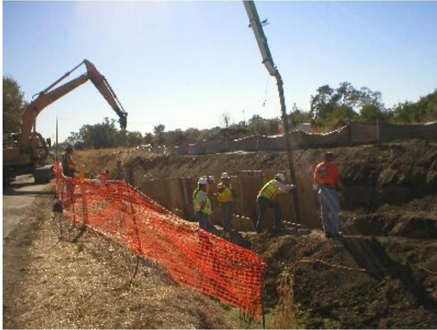
**Figure 1** – Concrete pour over the conduit installation within Drainage #30, October 6, 2005.
