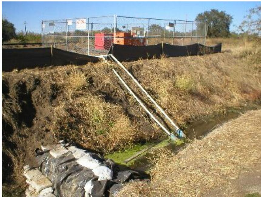
**Figure 2** – Dam and water pump system within Drainage #30 upstream of the work area, October 6, 2005.
