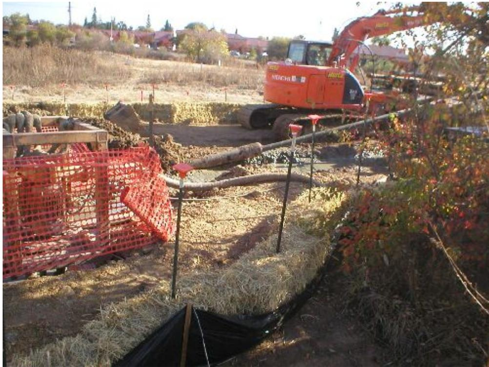
**Figure 4** - Bore rig. Note casing pipe around the rod and the flow of bentonite returns, November 21.
