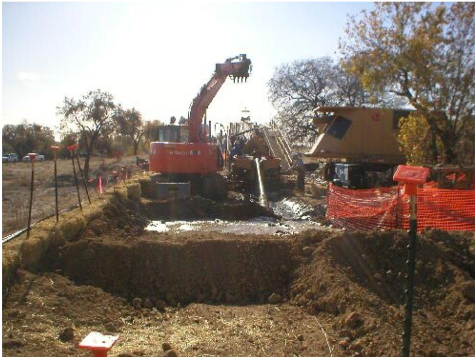
**Figure 2** - Bore rig setup, November 21, 2005.
