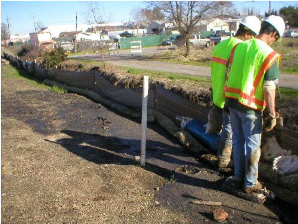
**Figure 2** – Crews placing sand bags at Seasonal Drainage #30, January 6, 2006.
