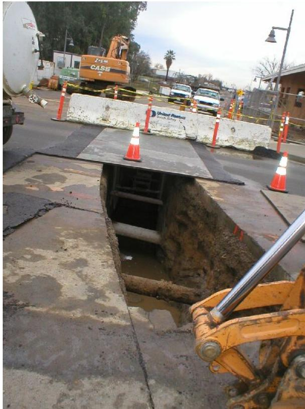
**Figure 2** – Trench and conduit installation within Rocklin Road, January 30, 2006.
