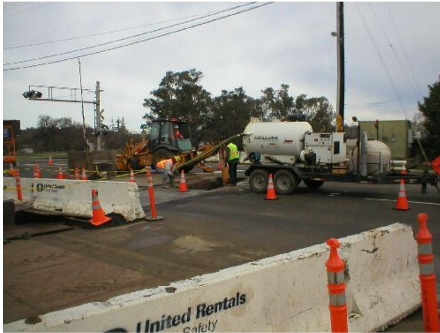
**Figure 3** – Crews using a vacuum truck to remove storm water from the trench within Rocklin Road, January 30, 2006.
