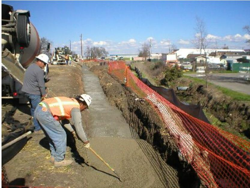
**Figure 3** – Thermal concrete pour adjacent to Drainage #30, February 16, 2006.
