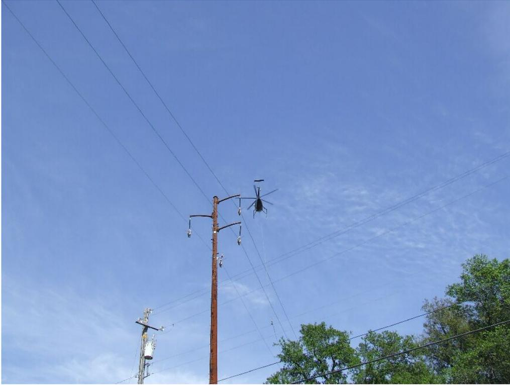
**Figure 1** – Wire-pulling between Del Mar Substation and Tower 9 using a helicopter, April 20, 2006.
