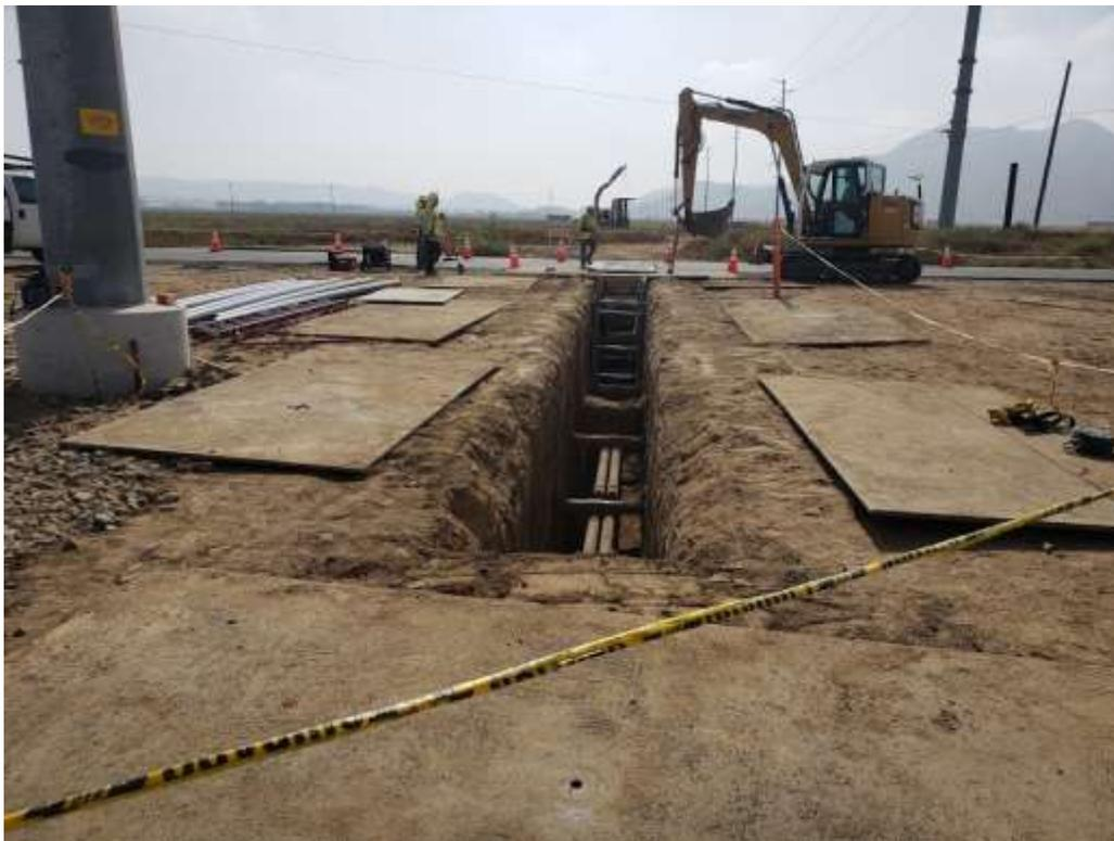
Photo 2 – Underground trenching and conduit installation under Menifee Road (June 26, 2019).
