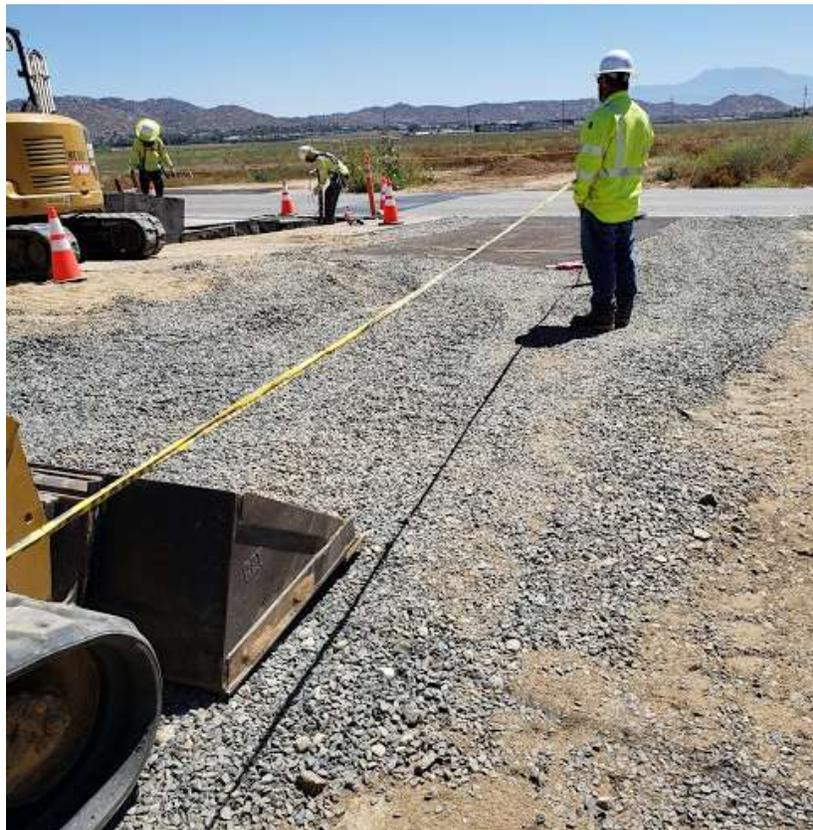
Photo 4 – SWPPP TC-1 required stabilized construction entrance on west side of Menfee Road near Valley Substation (July 2, 2019).
