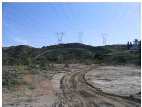
**Figure 4:** Access Road B leading to soil disposal site after grading through retention basin. This roadway was proposed on project maps to be used with no improvement.
