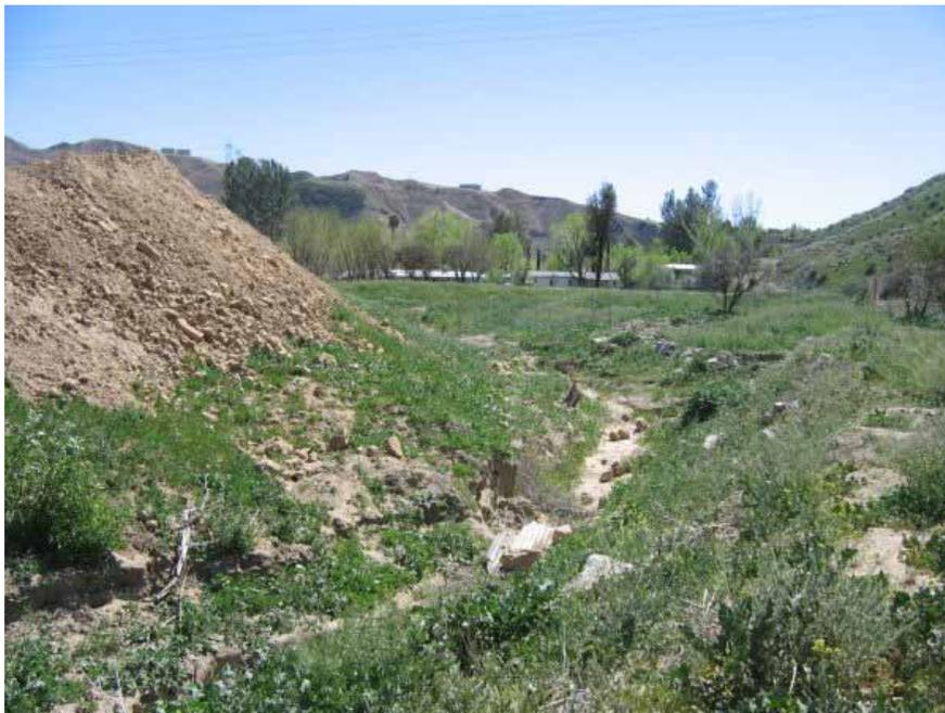
**Figure 2:** Soils from the excavation work at Tower 25 were used to build up earthen berms immediately adjacent to a dry drainage at the disposal site. Some material had slid into the channel, a Project Memorandum was issued by the CPUC EM for the non-compliance activity.
