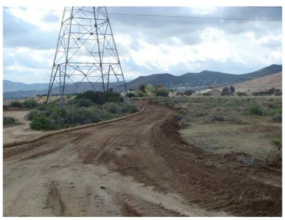
**Figure 4:** Grading of an access road for BMP installation at the Vincent Substation Expansion area.
