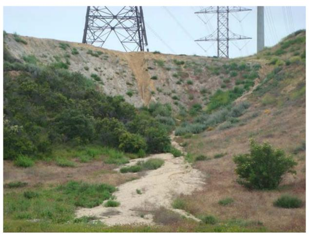
**Figure 1:** Erosion at Tower 9 in the City of Santa Clarita, Segment 1. A plan for repairs at this location is currently under review by SCE.
