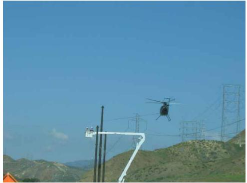
**Figure 1:** The installation of conductor wire between Shoofly poles 2-13 was completed using a helicopter. Once the sockline pulling cable was installed into each phase, the conductor wire was pulled back through the section and clipped in to each phase of the Shoofly pole.
