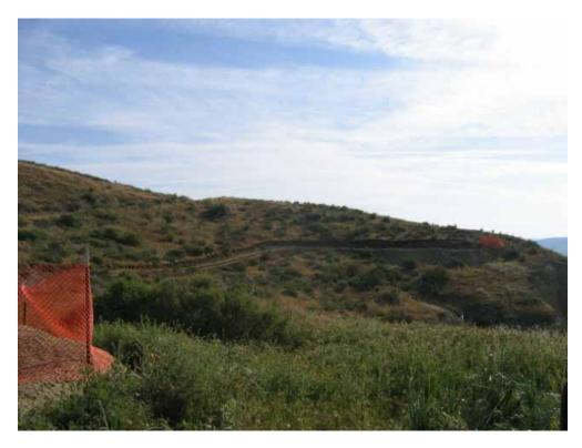
**Figure 2:** A new temporary road was constructed in order for pole setting equipment to safely access the Shoofly pole site 18. A Variance was approved by the CPUC for the change in road construction on April 3<sup>rd</sup>.
