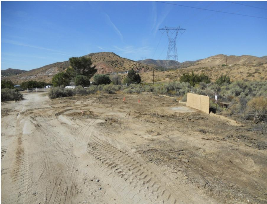
**Figure 2:** Covered foundation hole at TSP 5 and plywood to protect the adjacent drainage, Segment 5.
