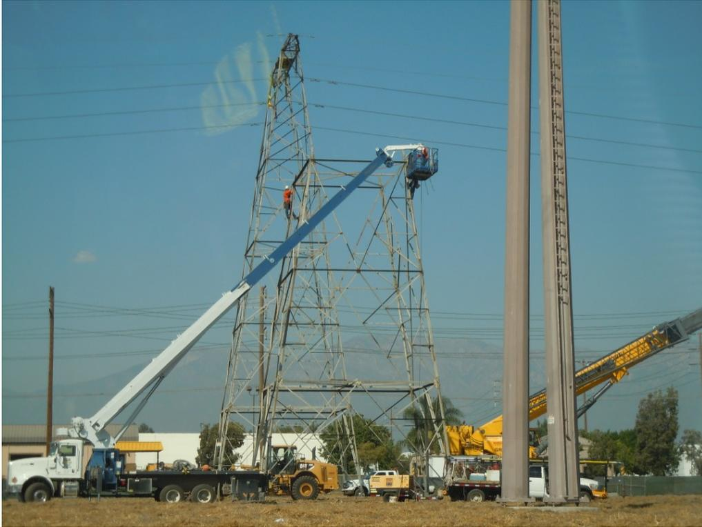
**Figure 3:** A Wilson crew works to remove tower M0-T3 in the City of Chino, Segment 8 Phase 2.
