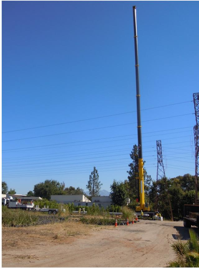
**Figure 5:** An SCE crew prepares to set a riser pole, Segment 7 66 kV.
