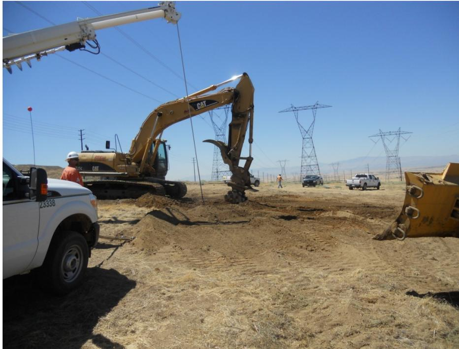
**Figure 1:** H&H Grading installed snubs in the wire set-up site between Towers 15 and 16, for upcoming wire stringing activity, Segment 4.
