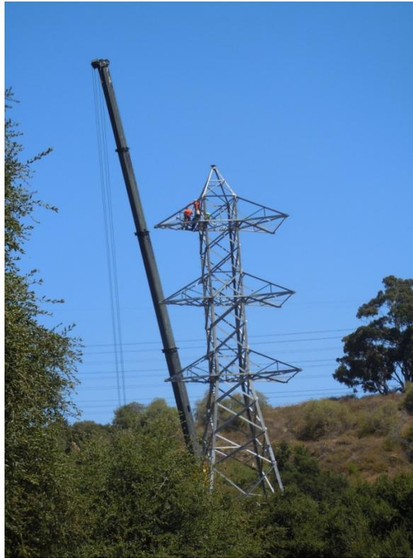
**Figure 7:** Crews build a tower within the PHLNHA, Segment 8 Phase 4.
