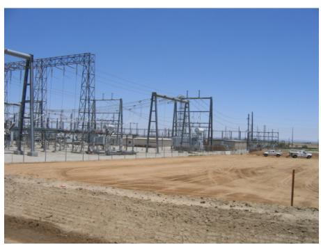
**Figure 2:** Grading of a portion of the Antelope Substation Expansion Area has been completed. Once the copper grounding is installed, rock will be brought in and the area will be fenced.
