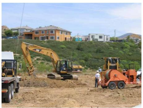
**Figure 2:** At Wire Stinging Site 9, near Haskell Canyon Road, crews began to remove the de-energized 220 kV lines.
