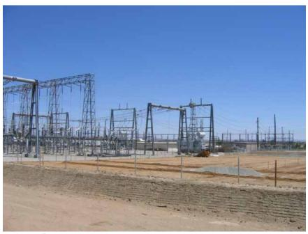
**Figure 5:** At the Antelope Substation, rock was delivered and fencing was installed surrounding the expansion area.
