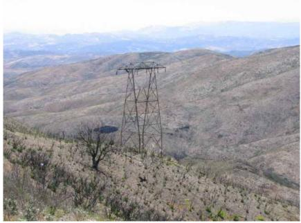
**Figure 3:** A 66 kV tower in the ANF (Section 2) was noted to have been vandalized by trespassers removing the copper conductor. SCE will seek approval from the ANF to remove the conductors prior to the issuance of the Section 2 SUP.
