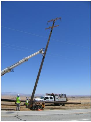
**Figure 5:** The 12 kV distribution poles set along Avenue K.
