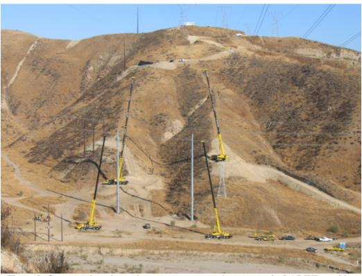
Figure 2: Cranes and steel guard structures were used to protect the LADWP corridor during wire removal over Haskell Canyon.
