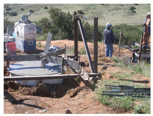
**Figure 2:** Pouring foundations in Segment 2.
