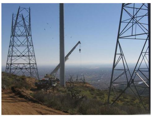
**Figure 3:** Steel assembly at Tower 28 in Segment 2.
