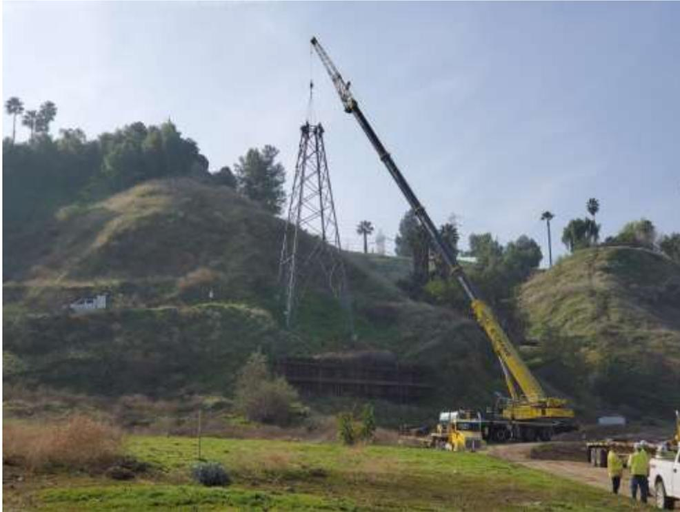
Photo 1 – Tower wreck-out at Construction Area 2N30, Segment 2 (January 14, 2020).
