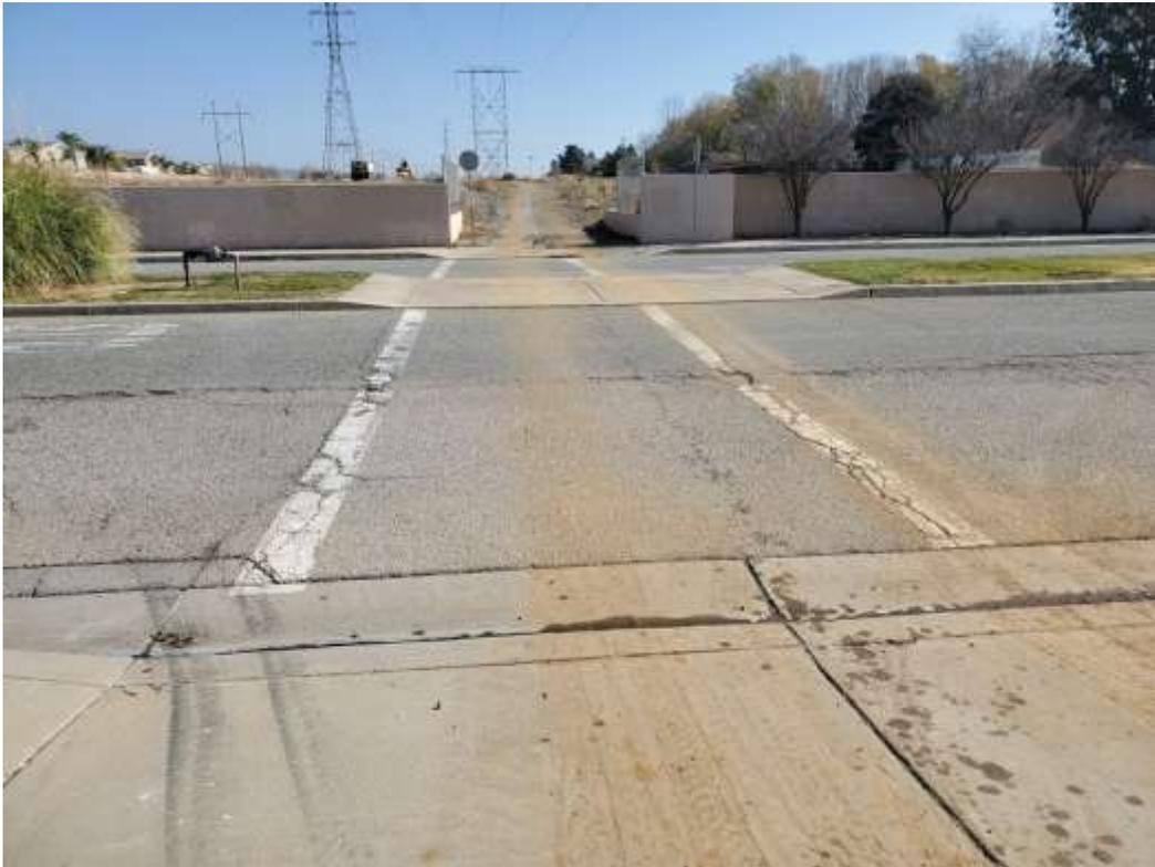
Photo 4 – Track-out on paved public road between Construction Areas 4X29 and 4X30, Segment 4 (January 13, 2020).
