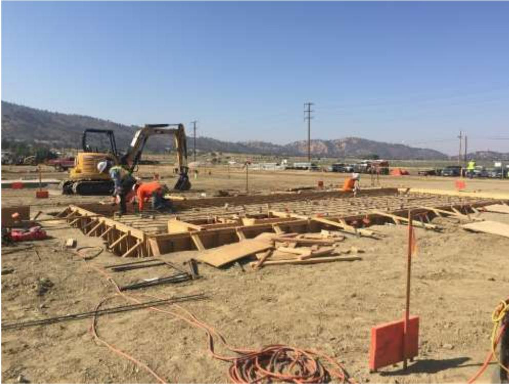
Figure 1 – Construction crews began foundation construction inside the Banducci Substation.
