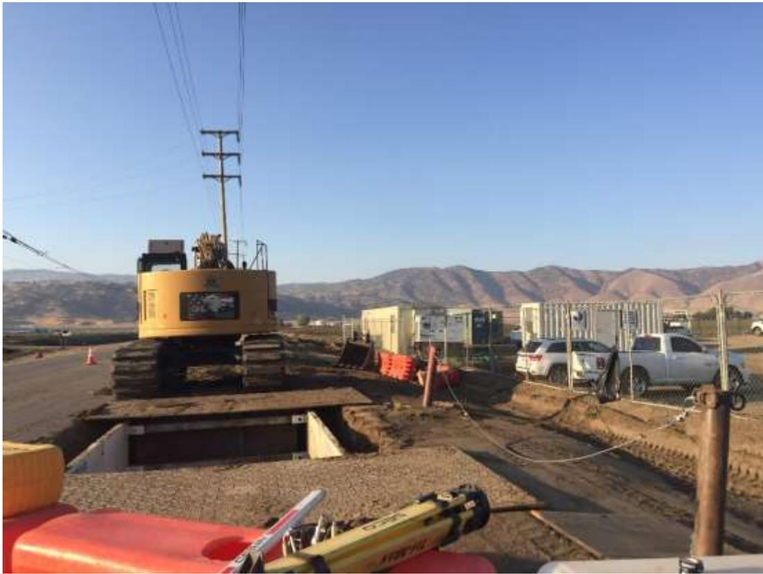
Figure 3 – Vault excavation for the underground subtransmission work along Pellisier Road.
