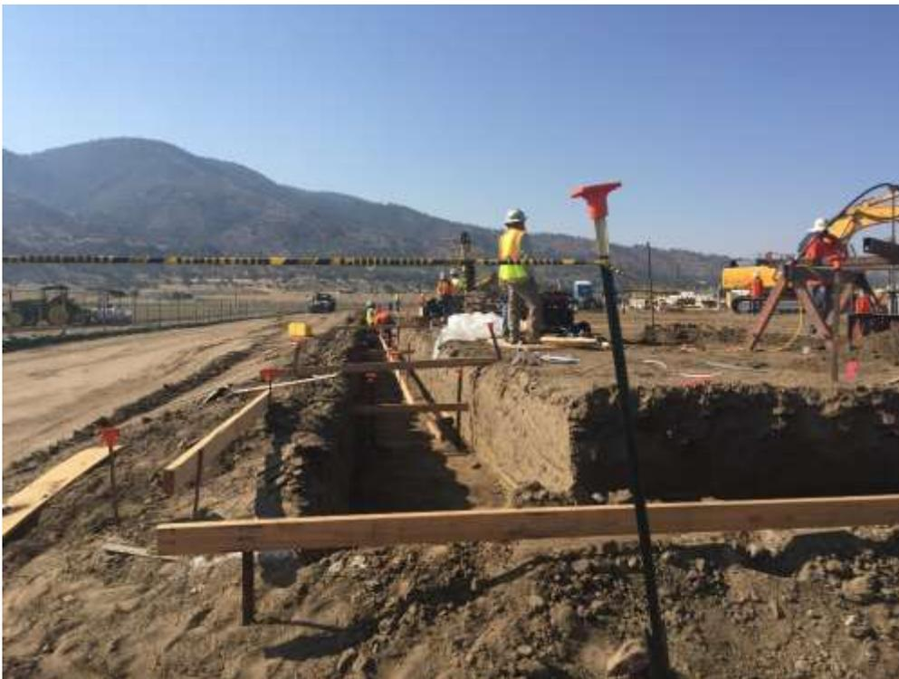
Figure 2 – Trenching for the perimeter wall foundation at the Banducci Substation.
