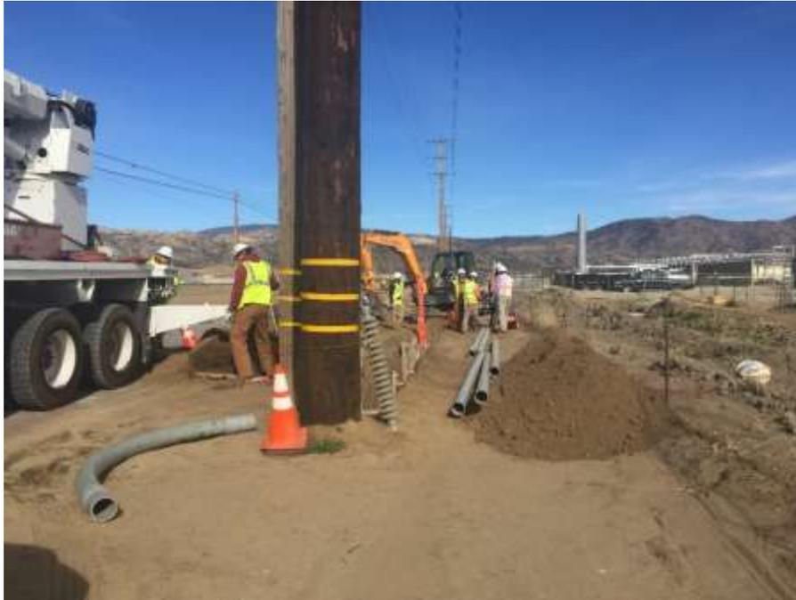
Figure 1 – Henkels and McCoy continue with trenching and conduit placement along Pellisier Road.
