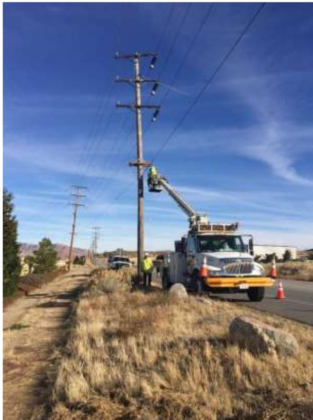
Figure 2 - Telecom crews installing fiber on existing poles along Highline Road, Route 1.
