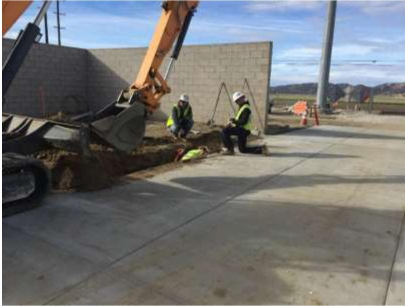
Figure 1 – Henkels and McCoy conducting trenching and conduit placement for the Substation driveway gate.
