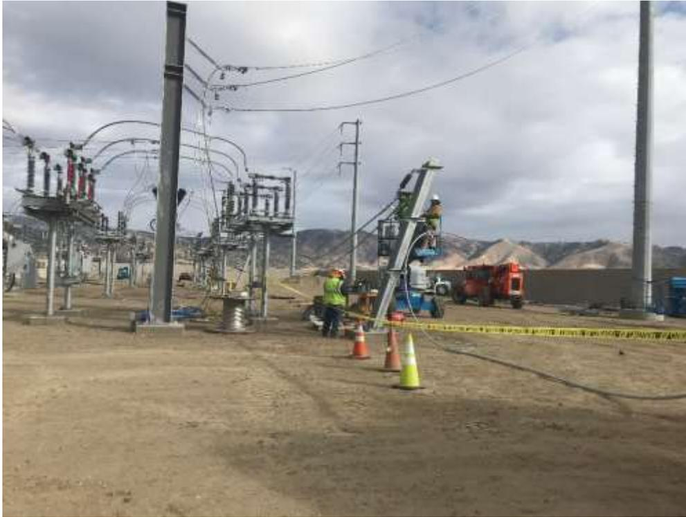
Figure 1 – Henkels and McCoy crew installing jumpers on the 66 kV rack.
