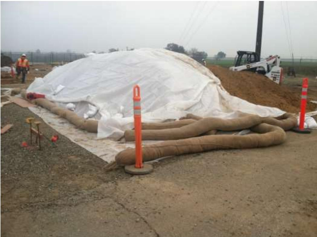
Figure 6 – SWPPP BMPs were installed to control runoff and protect stockpiled soil. View southeast, 12/10/14.
