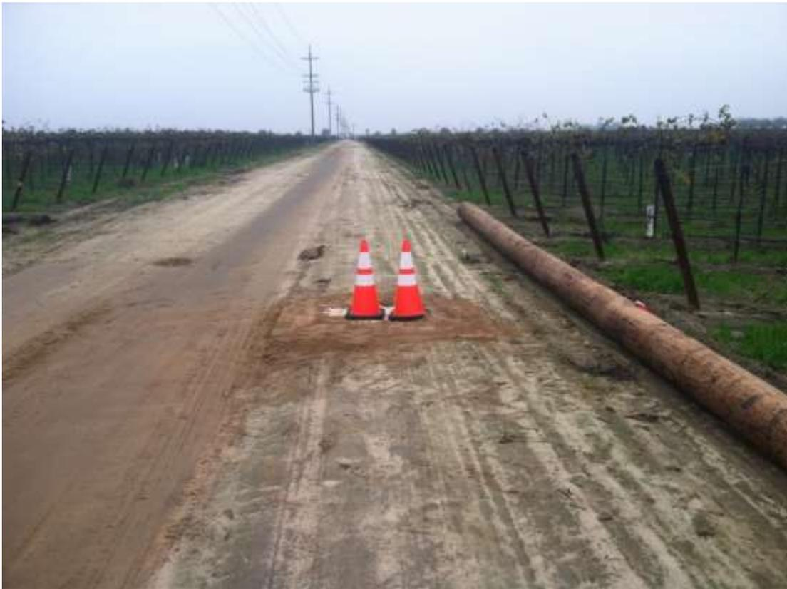
Figure 7 – Augered holes were securely covered at the end of the day. View south, 12/10/14.
