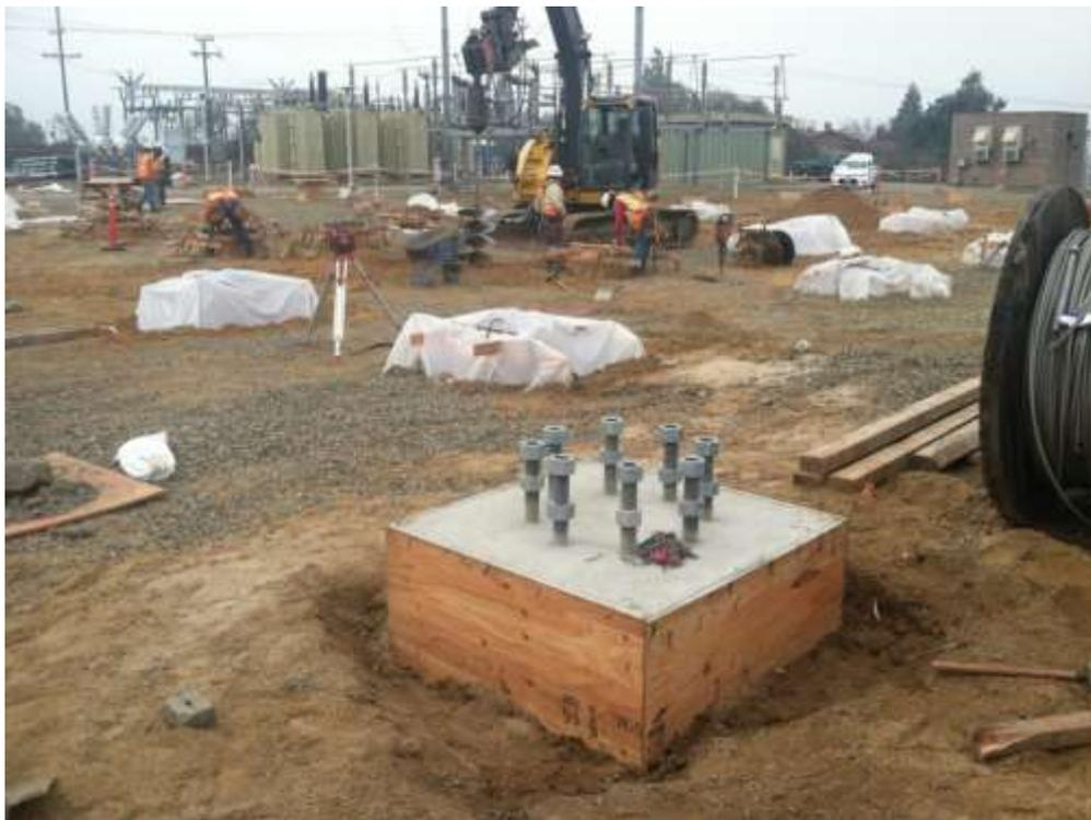
Figure 2 – Augering, trenching, and installation of concrete foundations occurred at the Cressey Substation during the subject week. View northwest, 12/10/14.
