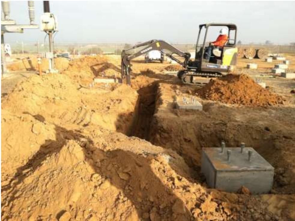
Figure 1 – Trenching occurred at the Cressey Substation during the subject period.
