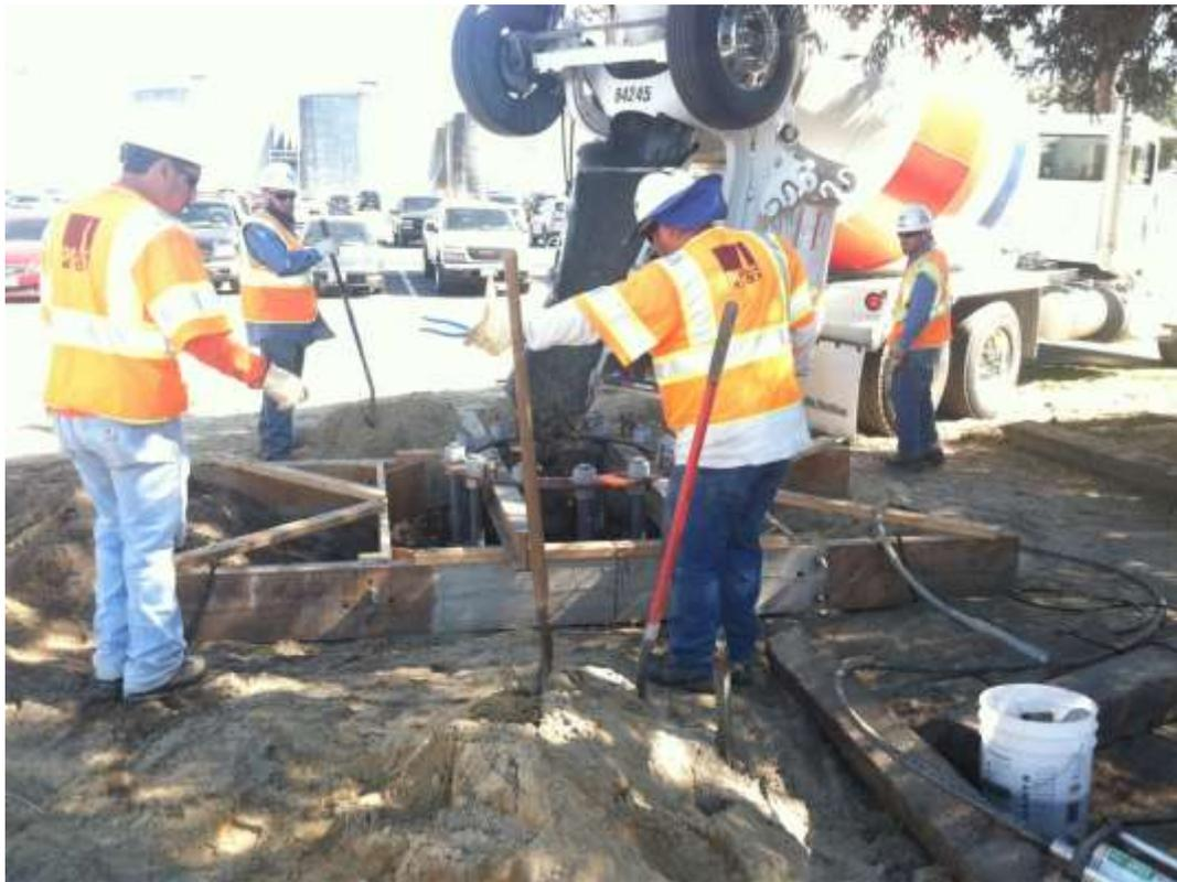
Figure 5 – Crews pour concrete for a TSP foundation adjacent to the Gallo Substation.
