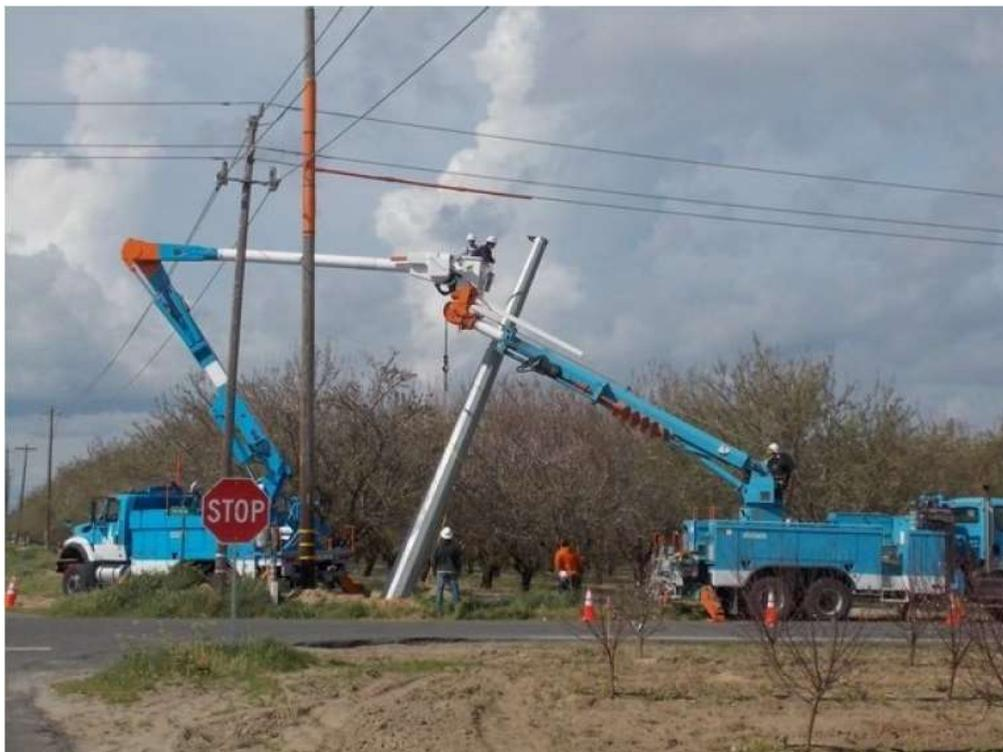
Figure 2 – Crews installed strain pole at the corner of Robin Avenue and Magnolia Avenue. View northwest. (Photo provided by PG&E).
