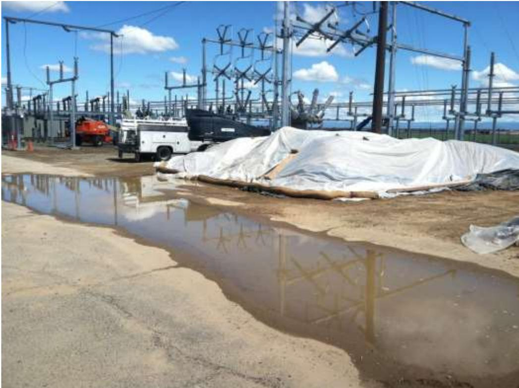
Figure 3 – Erosion control devices continue to be maintained in work areas and performed appropriately during a recent rainstorm. View northeast, 04/08/15.
