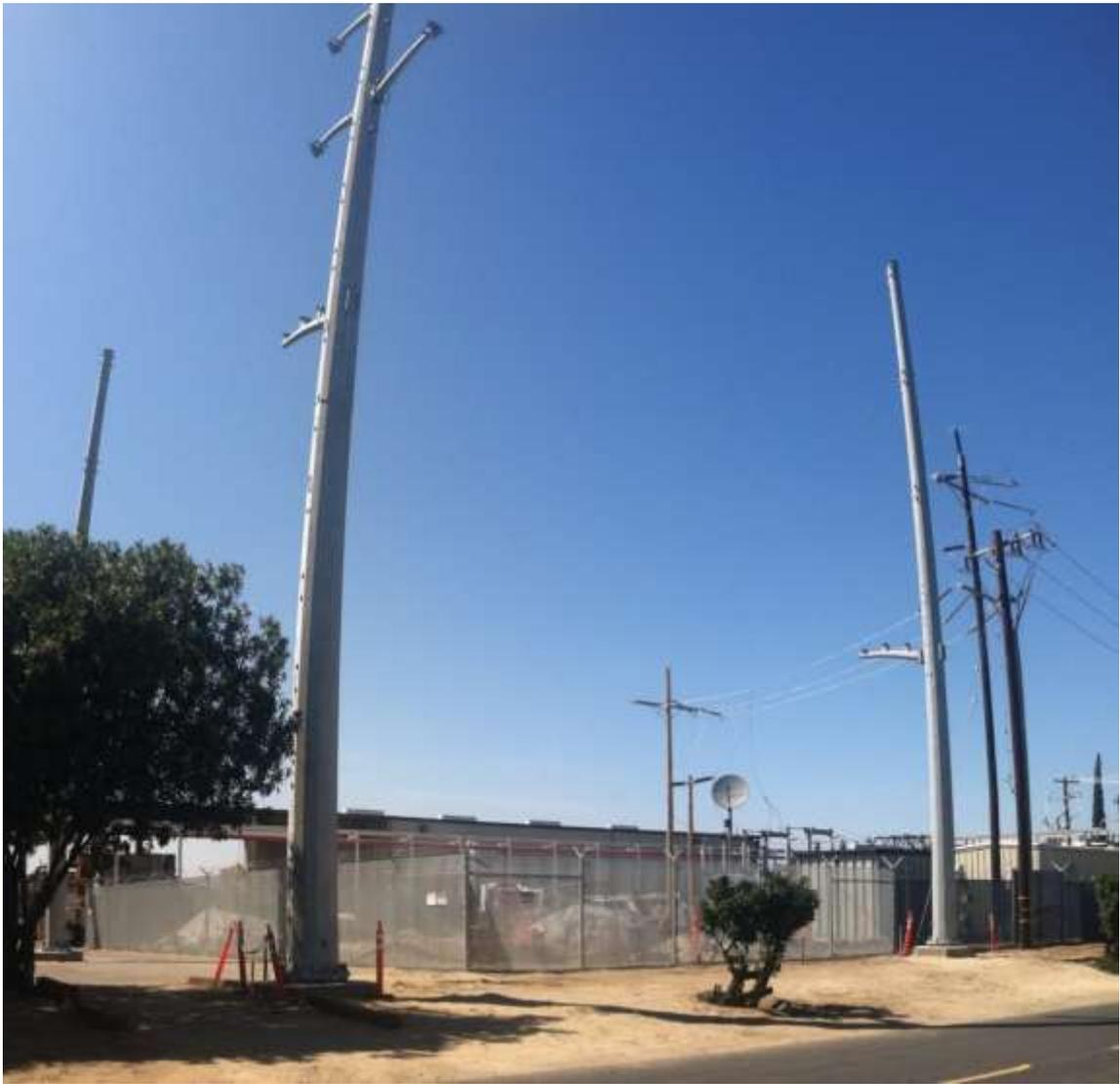
Figure 4 – Three TSPs and a VSAT dish were installed at the Gallo Substation during the subject period. View northwest, 04/15/15.
