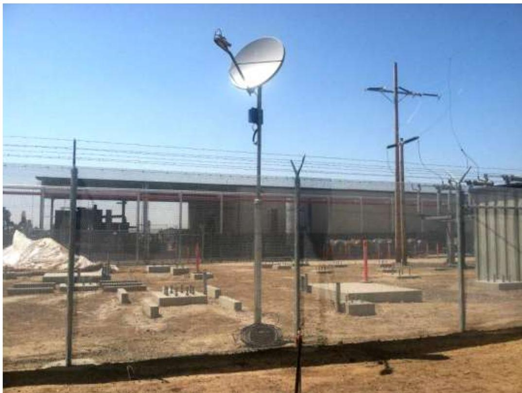
Figure 3 – Conduit installation and trenching were mostly complete at the Gallo Substation during the subject period. View northwest, 5/4/15.
