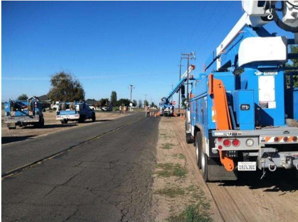
Figure 2 – Crews augered holes and set poles along the alignment during the subject period. View west (Photo provided by PG&E).
