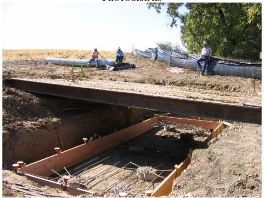
**Figure 1** – Bridge foundation work on south side of Sand Creek. September 20, 2007.
