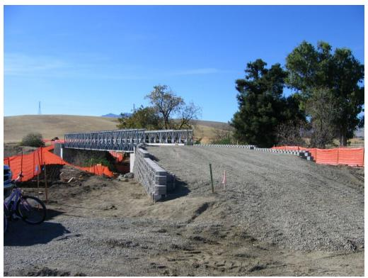
**Figure 1** – Keystone wall on either side of bridge over Sand Creek completed, November 14, 2007.
