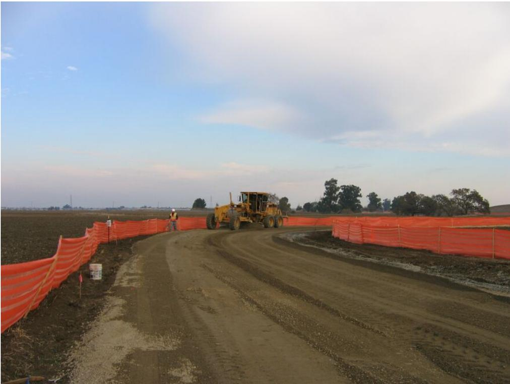
**Figure 2** – Final grading and compacting of access road to substation, December 12, 2007.
