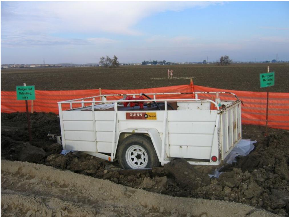
**Figure 3** – Designated refueling area at substation site with secondary containment, December 12, 2007.
