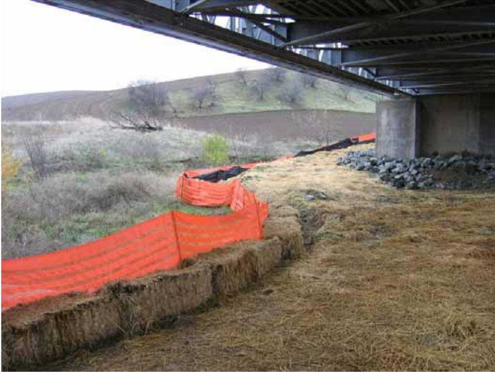
**Figure 1** – Restoration and erosion controls under Sand Creek Bridge, January 9, 2008.
