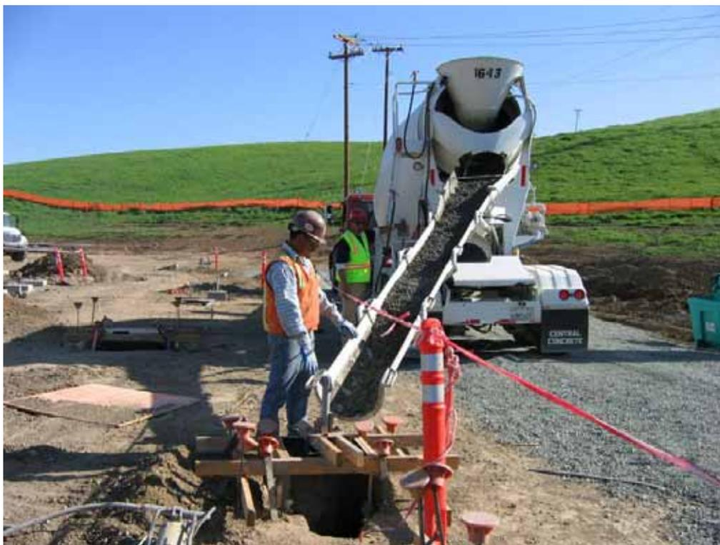
**Figure 4** – Pouring cement into pier holes, March 21, 2008.
