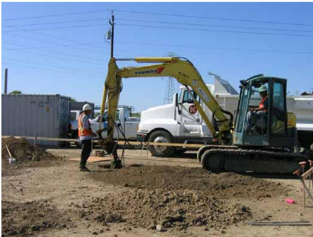
**Figure 3** – Crews drilling pier holes at the substation site, March 21, 2008.
