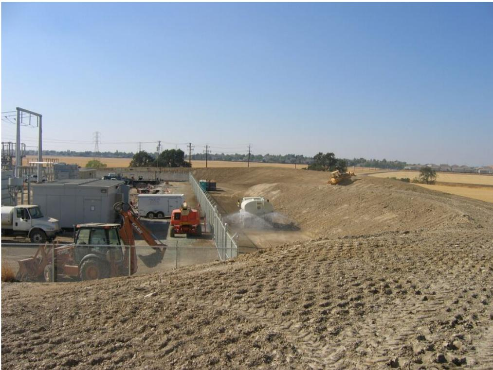
**Figure 4** – Earthen berm being built on the east side of the substation, June 24, 2008.
