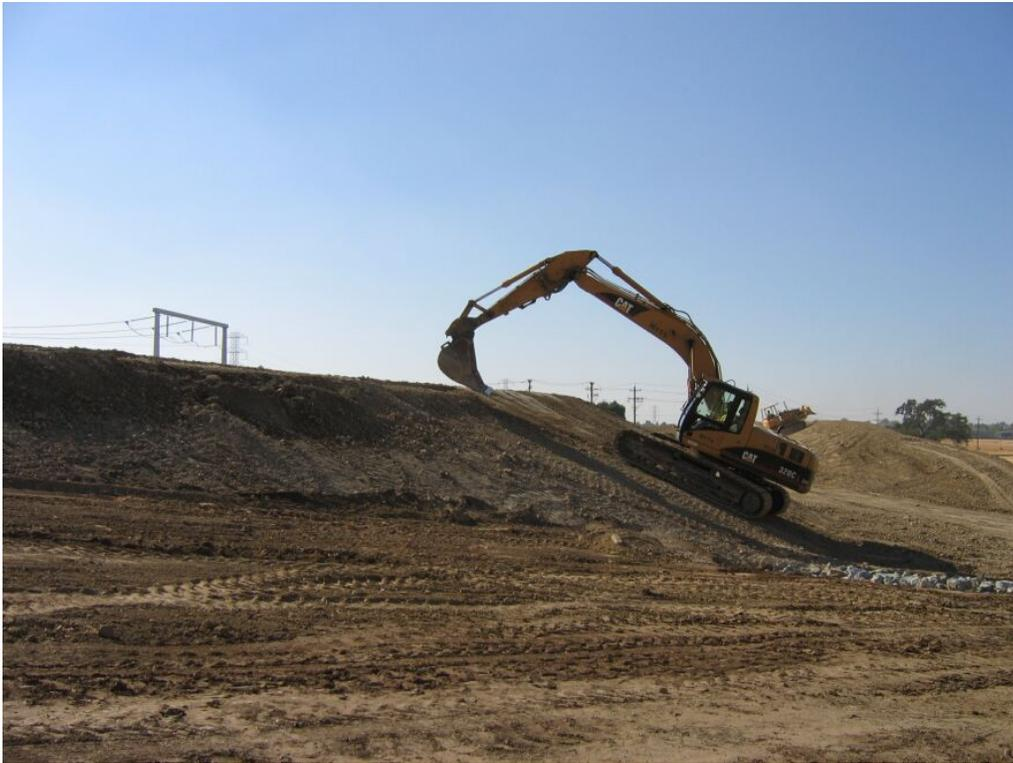
**Figure 3** – Earthen berm being built up around the outside of the substation, June 24, 2008.
