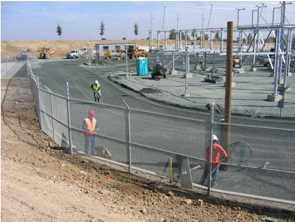
**Figure 2** – Crews preparing gravel for paving inside the substation, October 29, 2008.
