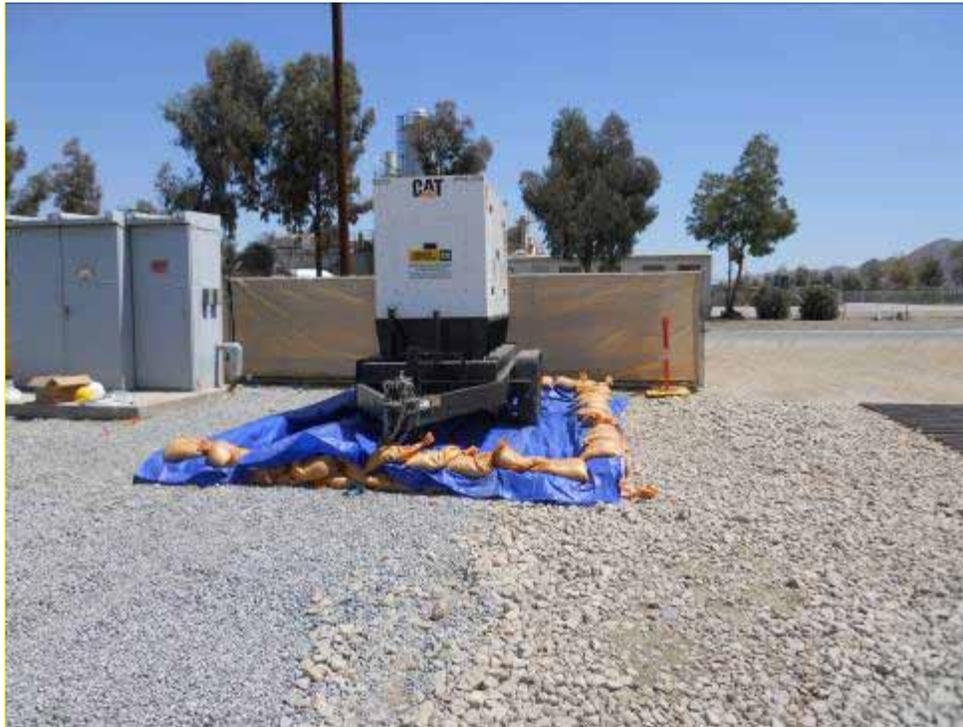
**Figure 8:** Example of secondary containment observed at Menifee Yard.
