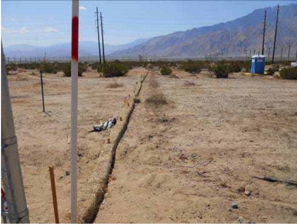
**Figure 3:** Installation of BMPs (straw wattles) at Devers Construction Yard.
