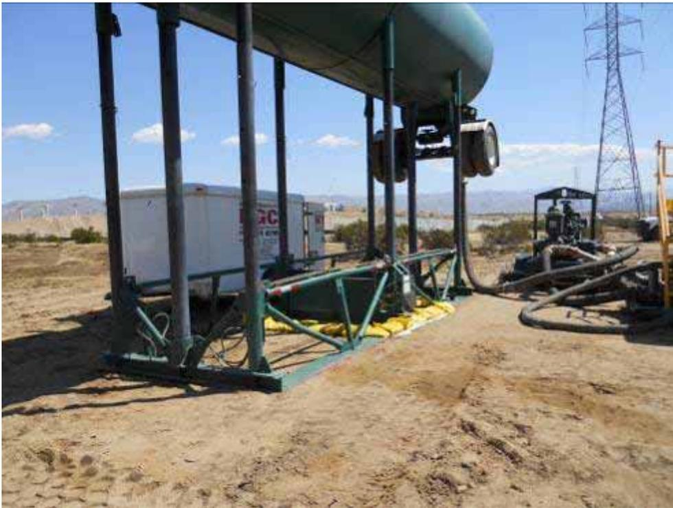
**Figure 8:** Example of secondary containment observed at Devers Yard.
