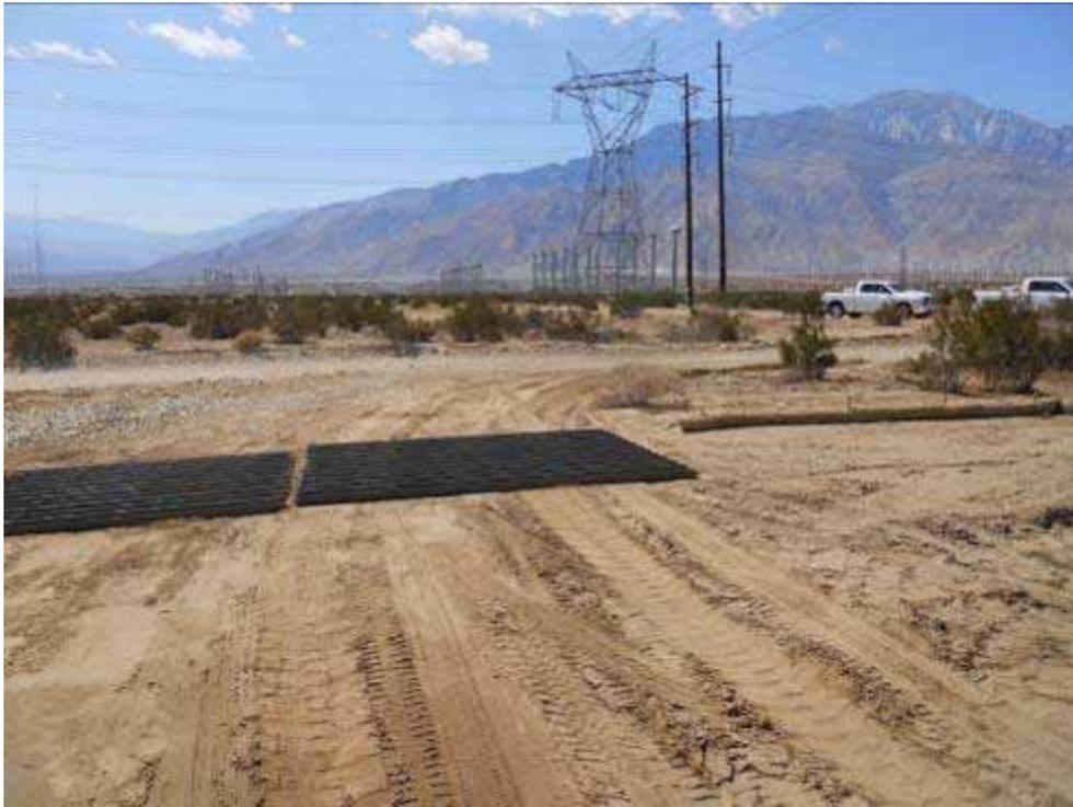
**Figure 7:** Tracker plates installed at entrance to Devers Construction Yard.
