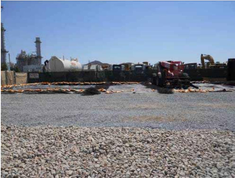
**Figure 9:** Secondary containment and protective netting being utilized at Menifee Construction Yard.
