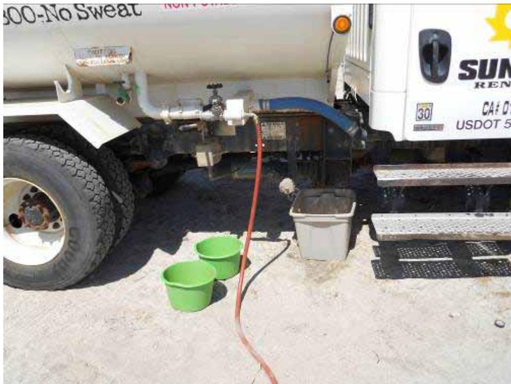
**Figure 8:** Drip pans installed underneath stationary water truck during exclusionary fencing activities.
