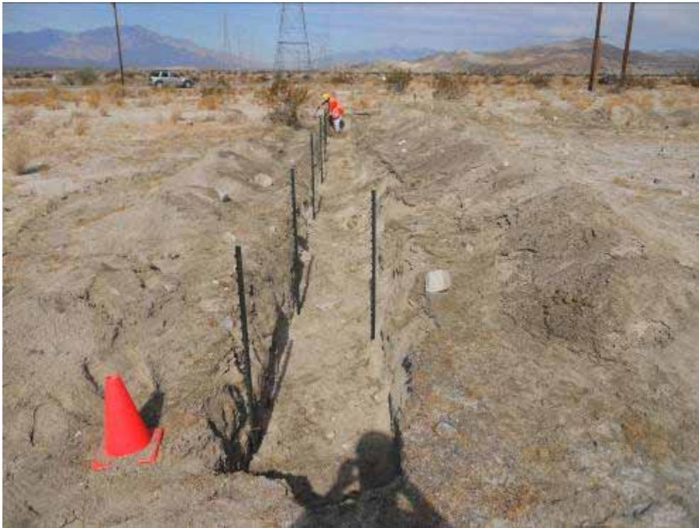
**Figure 7:** Trenching at exclusionary fencing locations.
