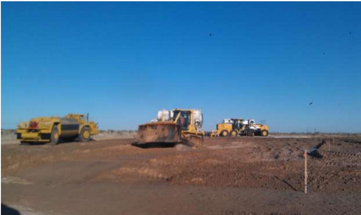
**Figure 4.** Grading of the laydown area within the CRS site (Photo Courtesy of Wilson Leung)
