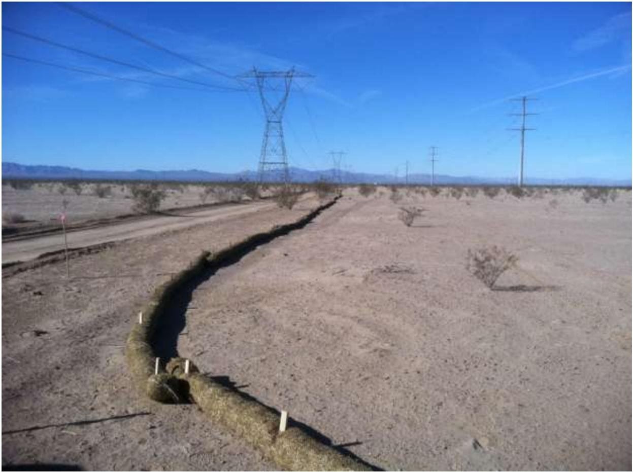
**Figure 2.** BMP installation along the access road to CRS from Wiley's Well Road.
