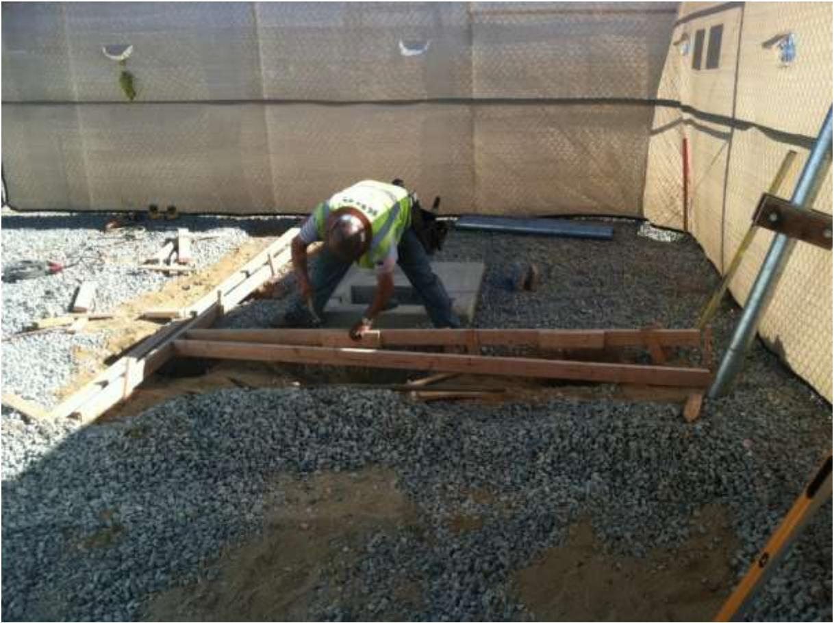
**Figure 7.** Preparation for auger drilling at the Devers Yard temporary power source.
