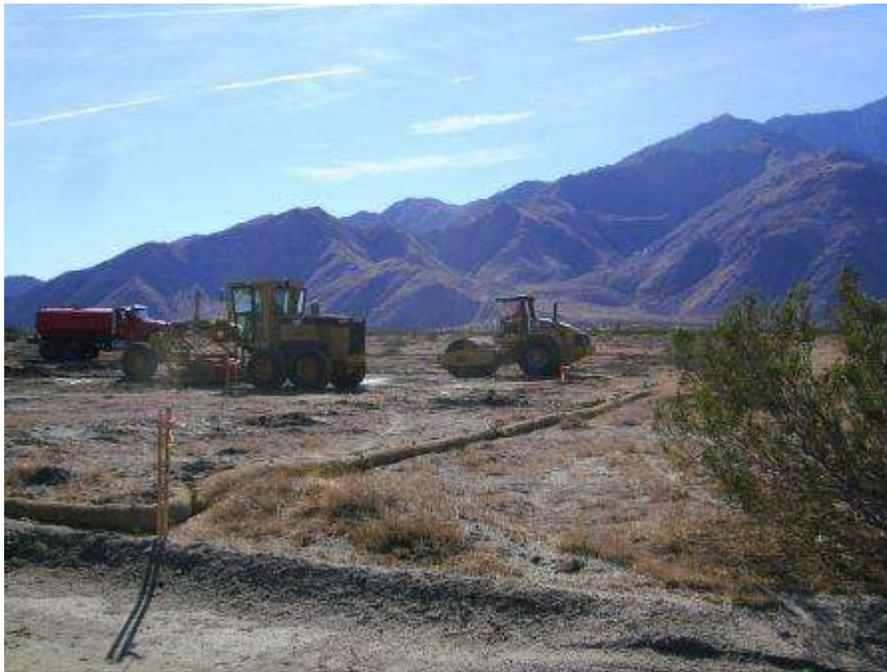
**Figure 4.** Grading of the crane pad at Tower 1024.
