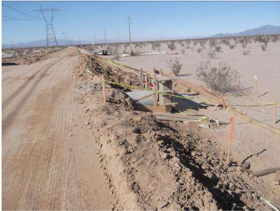
**Figure 7.** Culvert installation along CRS access road.
