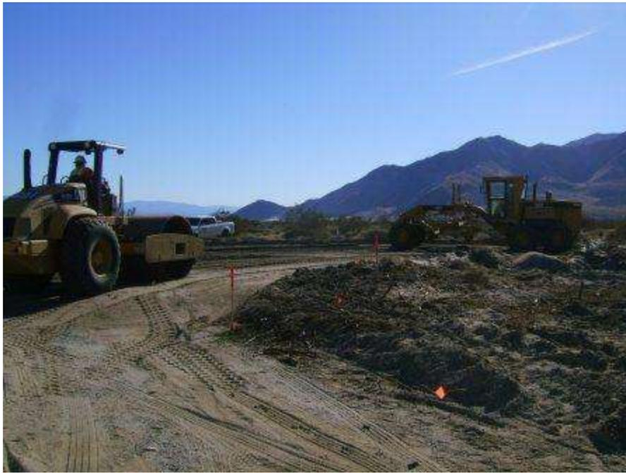
**Figure 3.** Spur road and crane pad grading at Tower 1029.
