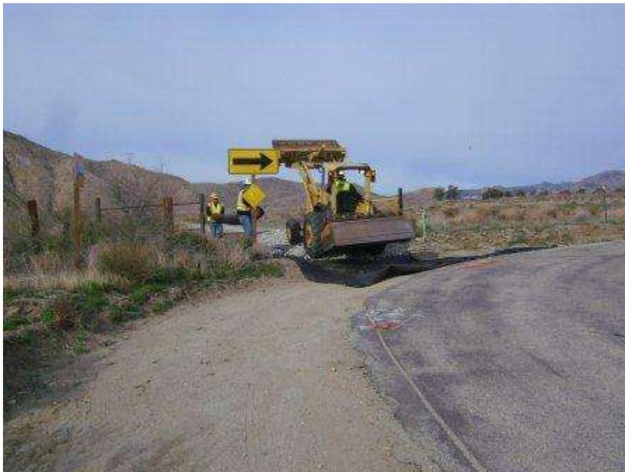
**Figure 4.** Gravel and rattle plate installation at the entrance to Tower 1062/R2.
